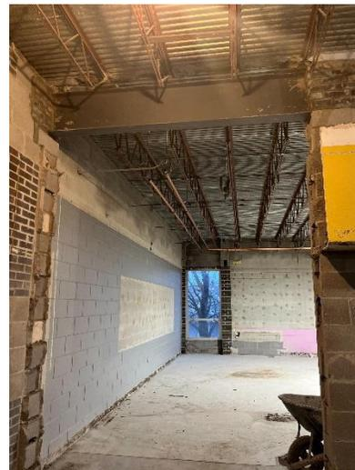
Steel Beams Installed for Bathrooms
