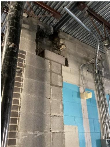
Bearing Plates Installed for Added Toilet Rooms
