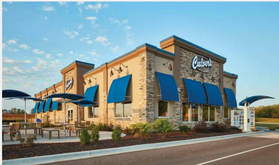
A common look of Culvers ↑
