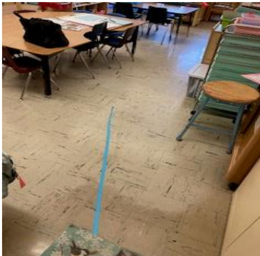
HA#12- Typical 9"x9" floor tile
